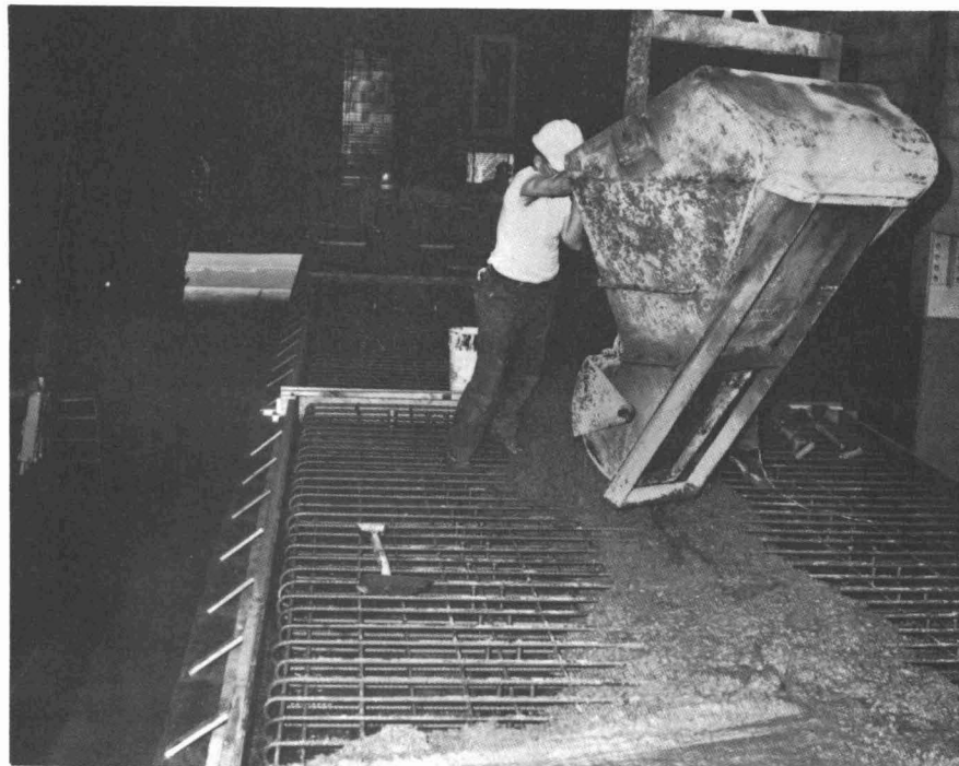
FIG. 4 - CONSTRUCTION OF COMPOSITE BEAMS
