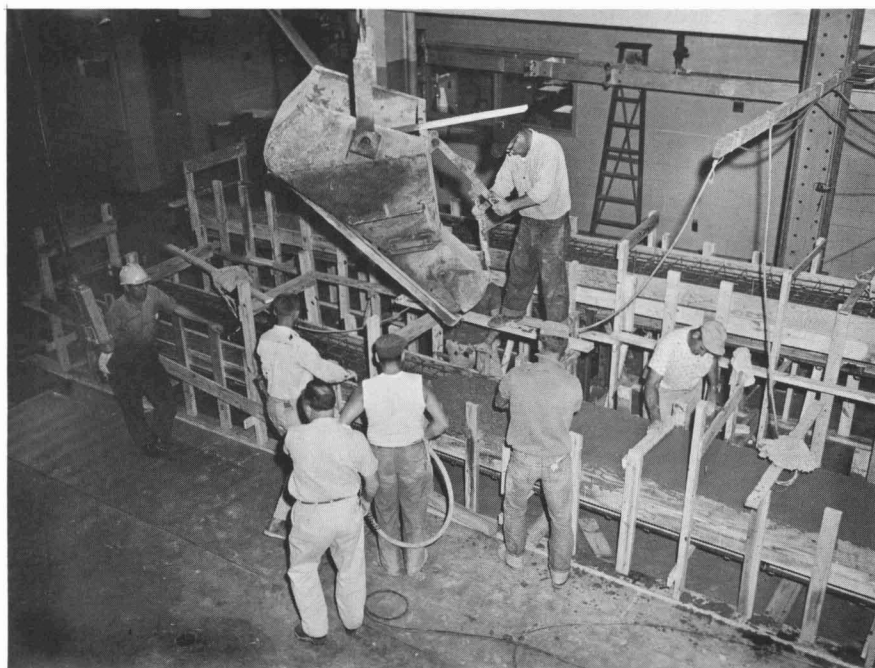
FIG. 8 POURING STAGE I CONCRETE, Re-I
