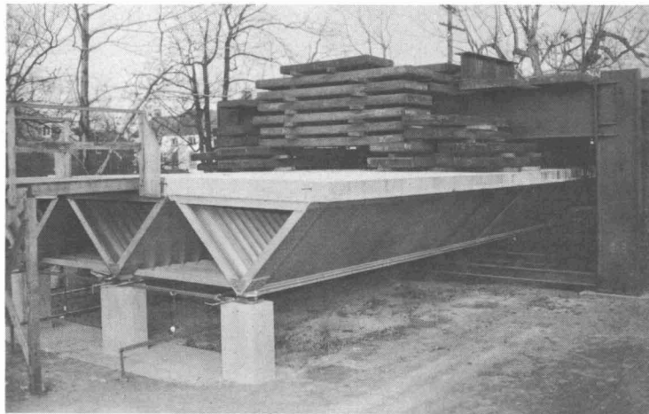
FIG. 9 STEEL SLABS PLACED ON BRIDGE DECK FOR DESTRUCTION TEST
