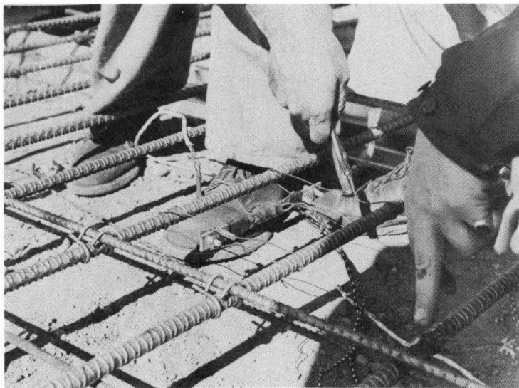
Figure 11 Placing of Concrete Strainometer in Test Panel
