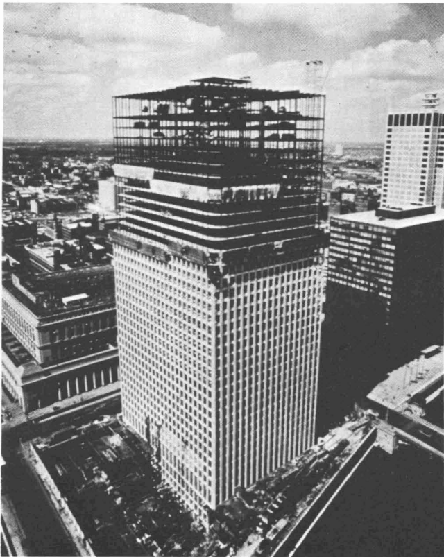
Fig. 25. Chicago building (Courtesy Engineering News Record)
