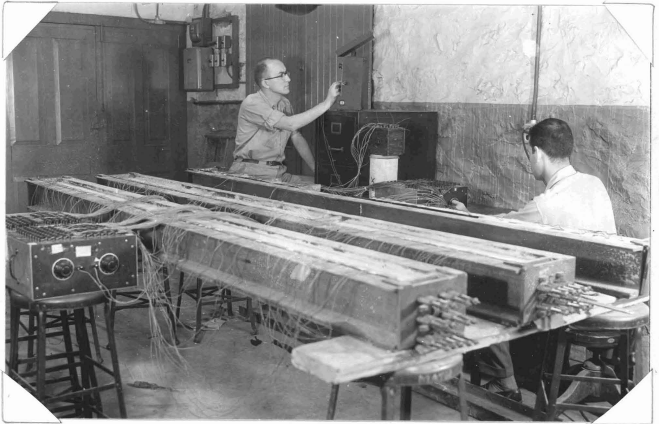
Figure (11) Actual Test Before Release of Prestress
