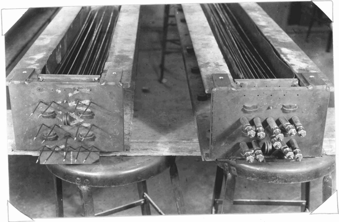
Figure (7A) End View of Two Forms Showing Threaded Wire Ends, Dead Ends, and Prestress- ing Devices
