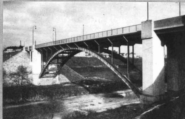
Fig. 9 - German All Welded Two-Hinged Arch Bridge
