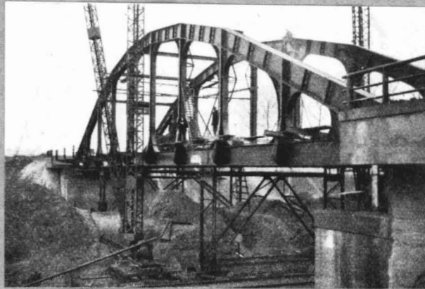
Fig. 8 - Photograph of the Vierendeel Bridge
