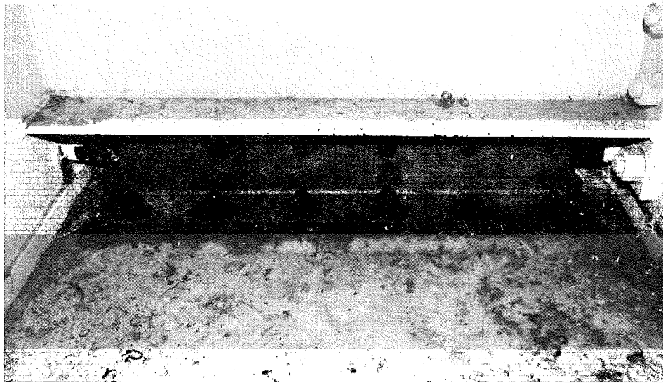
Fig. 21 Initial Retrofit Angles Attached to Diaphragm and Bottom Flange
