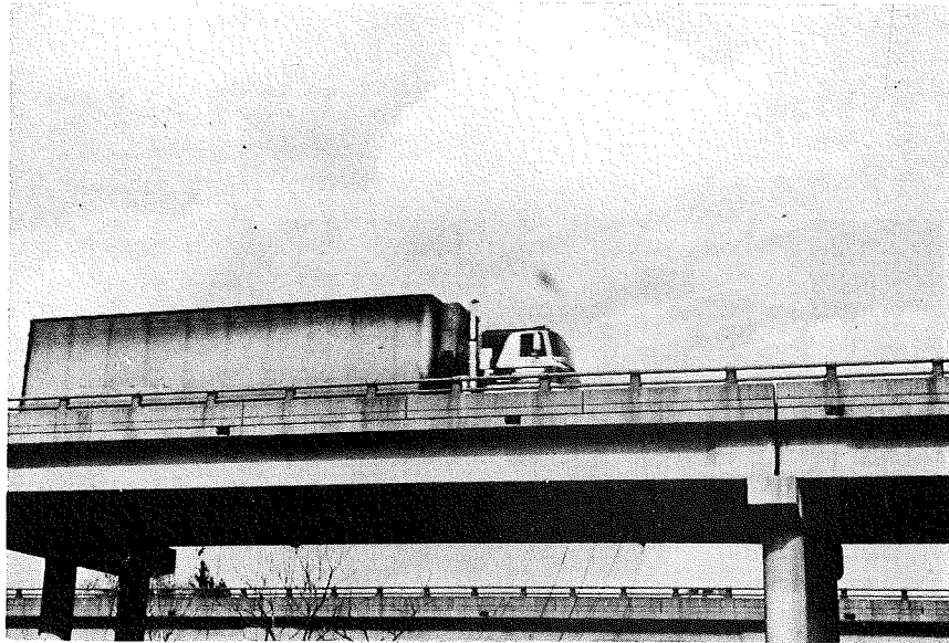
Fig. 14 Truck Crossing Immediately West of Truck Weighing Span
