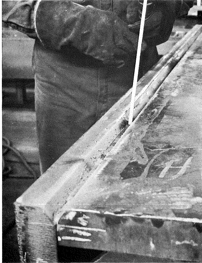
Fig. 13 Seal Weld Deposit on the Box Shape.
