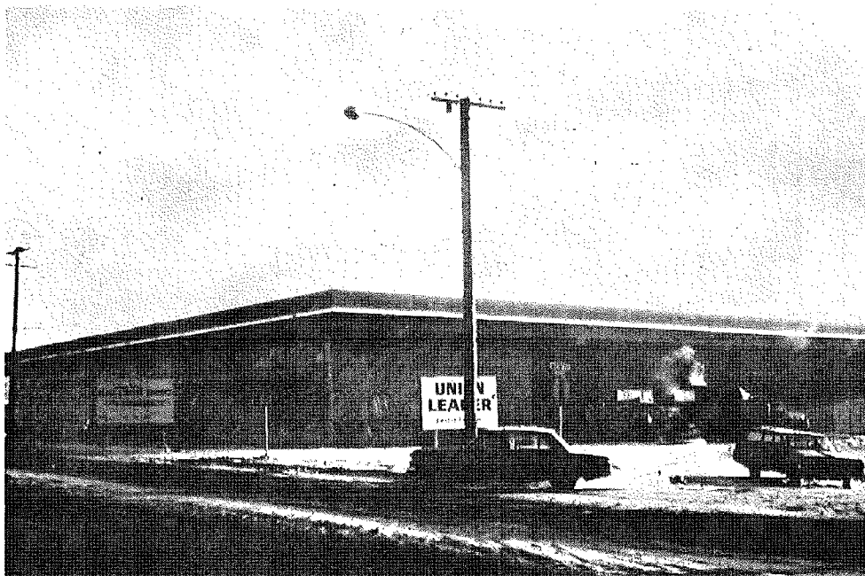
Fig. 40 Alaska Sales and Service Building, November, 1964
