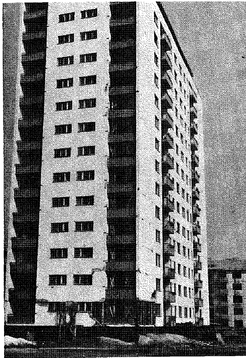
Fig. 24 Karpos Tower, March, 1965
