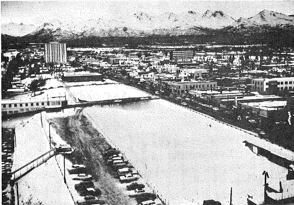
Fig. 38 Fourth Avenue Slide Area, November, 1964
