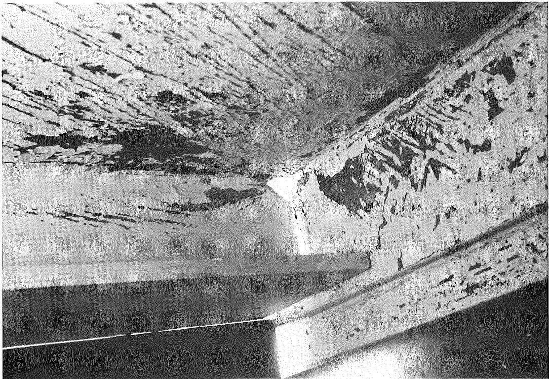
Fig. 4.21 Typical Stiffener Detail at Tension Flange (E2-T2)
