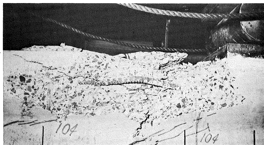
c. View of Failure Region
