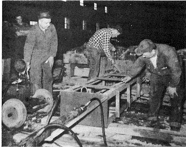
Fig. 8 Stressing of Individual Strands
