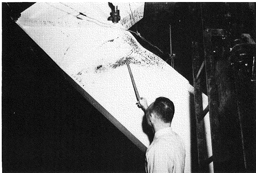
After the ultimate load on the connection was reached, local buckling appeared in the web and compression flange.
