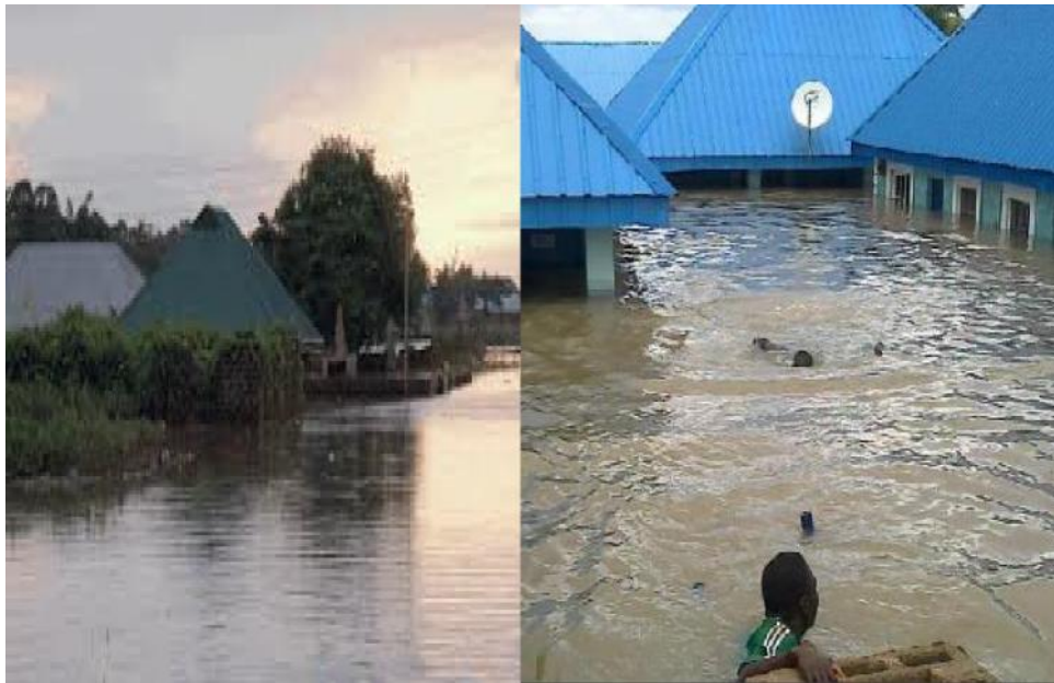
Figure 3.18 Evidence of Flooding North Central Region (Makurdi).
