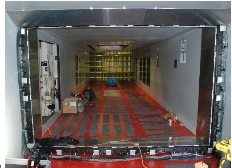
Forward fairing installed, routing of detector and source cabling on aft side (aft looking forward)
