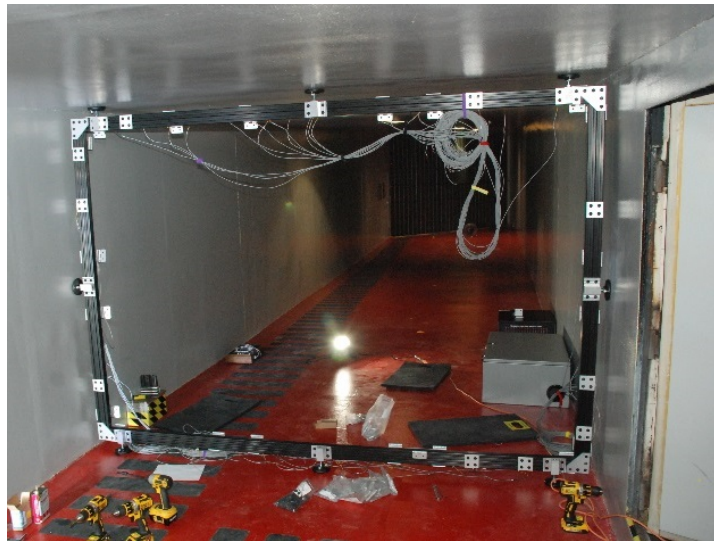
Frame mounted to tunnel walls (forward looking aft)
