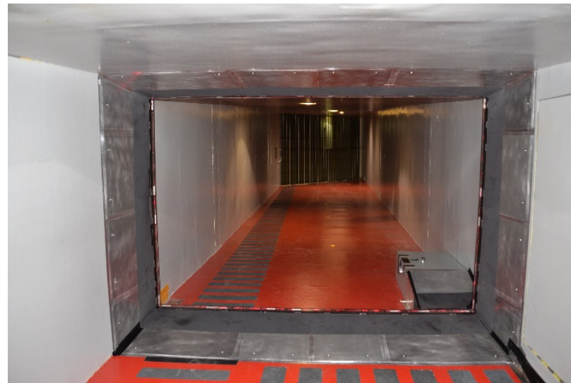
Final system installation (forward looking aft)
