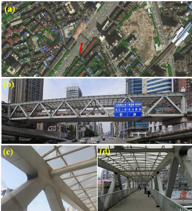
Fig. 3. Xima Road pedestrian steel bridge: (a) Baidu Map© view shows the pedestrian bridge and its vicinity; (b) elevation view; (c) connection detail between strut, top chord and diagonal chord; (d) longitudinal view.
