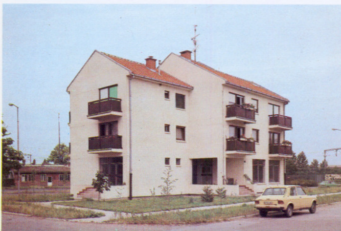
Fig. 17 Experimental (multi-family) dwelling in Novi Sad with commercial facility at ground floor
