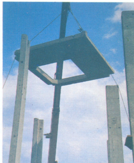
Fig. 10 Erection of staircase floor slab
