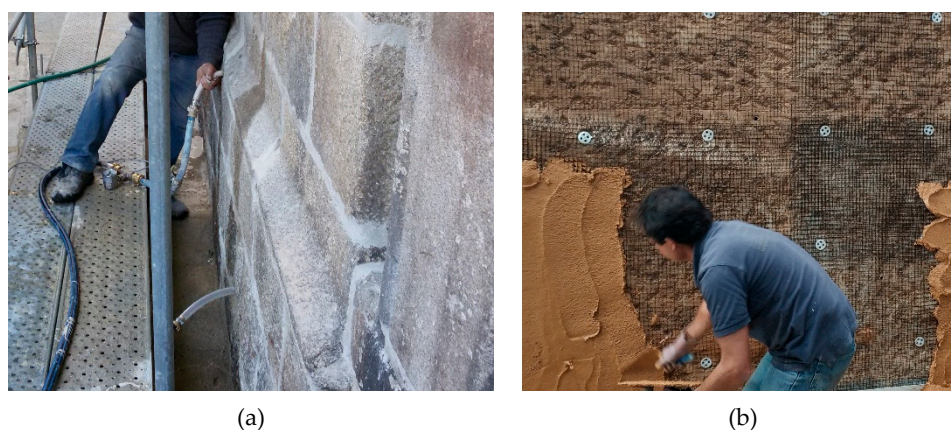
Figure 8. Examples of innovative strengthening solutions: (a) grout injection and (b) textile-reinforced mortar (TRM).
