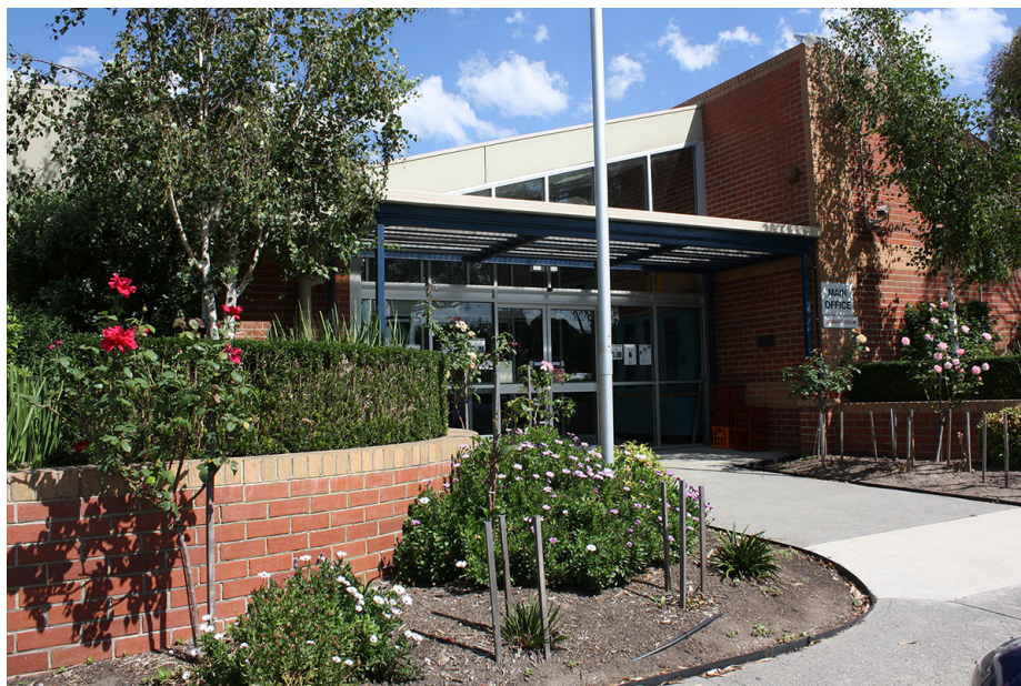
Figure 5. Main entrance of Hanworth Secondary College (Source: school website).
