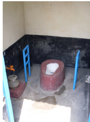
Toilet built for people with a disability in Dhaka, Bangladesh. Credit: Juliet Willetts
