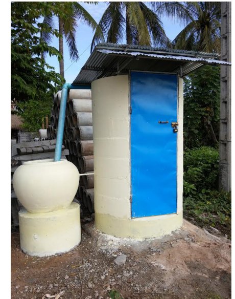
The Ring Shelter, a more basic and affordable alternative. Credit: iDE Cambodia
