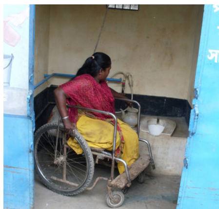
Toilet built for people with a disability in Dhaka, Bangladesh. Credit: Juliet Willetts
