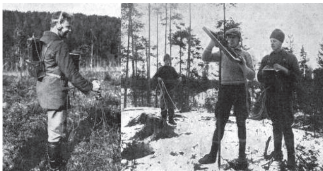
Figure 1: (left) An early Swedish equipotential mining survey, (right) Electromagnetic mining survey using the Sundberg method. Picture from Yearbook nr 17 of the Swedish geological survey (1923).
