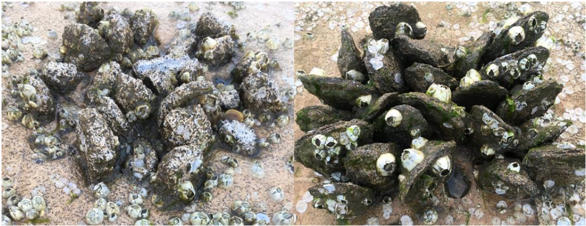
Figure 33. Substrates constructed with magnesium concrete mixture (left) exhibited greater rates of erosion than substrates constructed with standard concrete (right). Above photos taken at the time of the final data collection period (January 2019).
