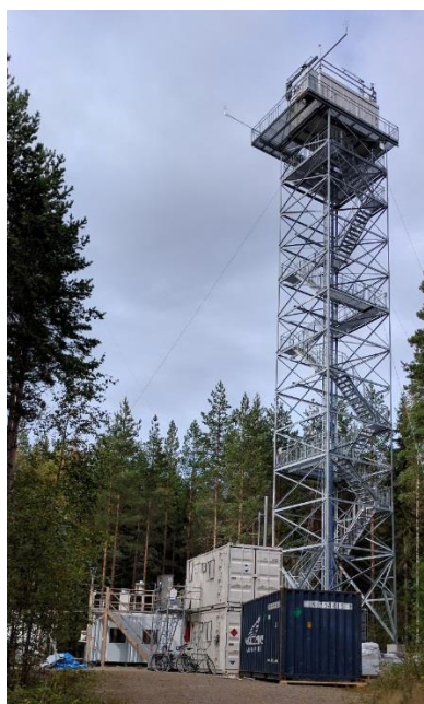
Figure 4.6 Photo of the MPIC measurement containers installed in place for the IBAIRN-2016 campaign, including 8.5 m common inlet for the instruments.
