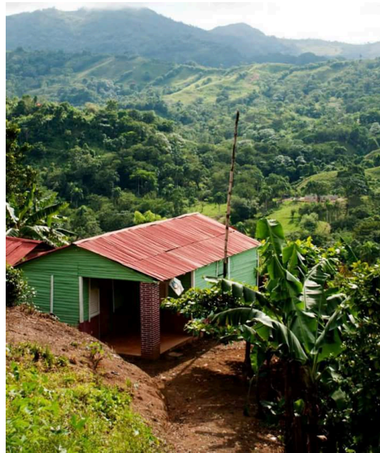
Figure 43 House in the Cibao countryside, Dominican Republic
