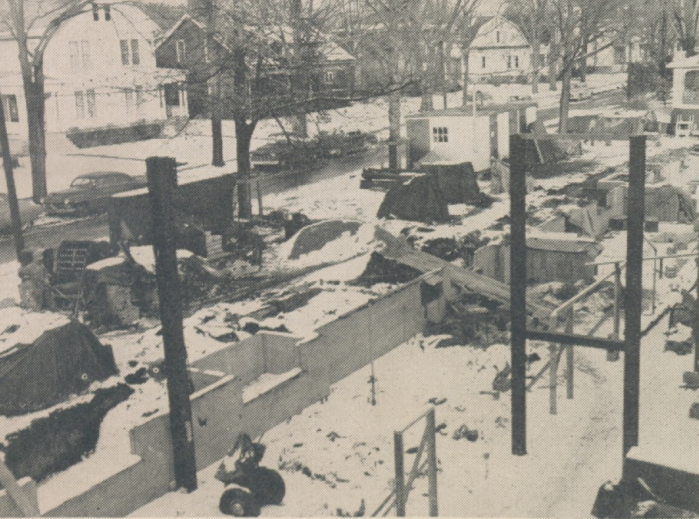
Construction is begun on Clements Hall.
