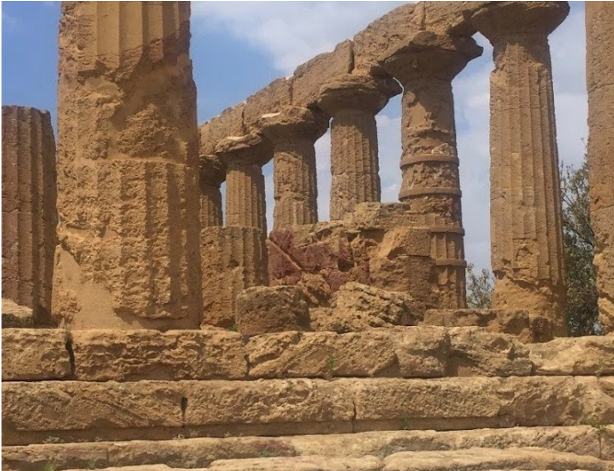
Figure 2.1: Discoloration on the Tempio di Giunone (Temple of Juno)- evidence of the fire set during the Siege of Agrigento. Agrigento, Sicily.
