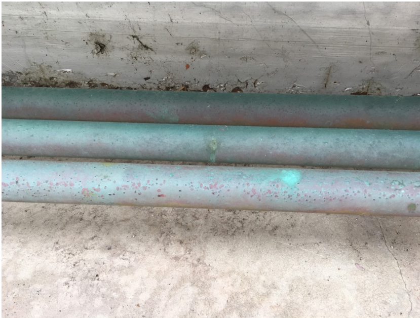
Figure 8: Desert House, Wellesley College Botanic Gardens, detail of blueish green pipes.
