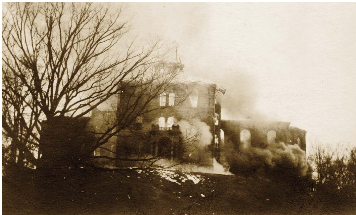
A view of the east end of College Hall in flames on March 17, 1914, at about 7 A.M.
