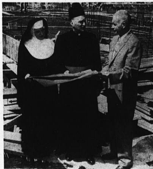
EARLY PLANNING: Joseph Smith, right, stands on foundations of St. James Hospital discussing blueprints with Sister Patricia Aidan, C.S.J., administrator, and Msgr. Thomas M. Reardon, pastor of St. James parish. Hospital was dedicated in early 1961.
