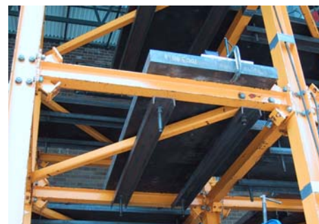
FIGURE 3: PHOTOGRAPH SHOWING MASS PLACEMENT.
