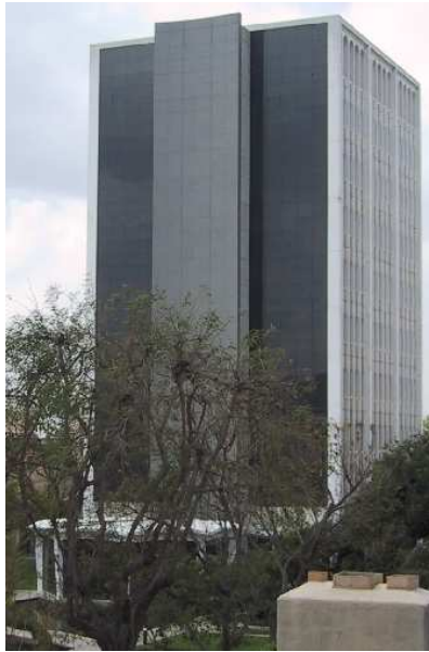
Figure 1. Robert A. Millikan Memorial Library: View from the Northeast. The two dark colored walls in the foreground comprise the East shear wall.
