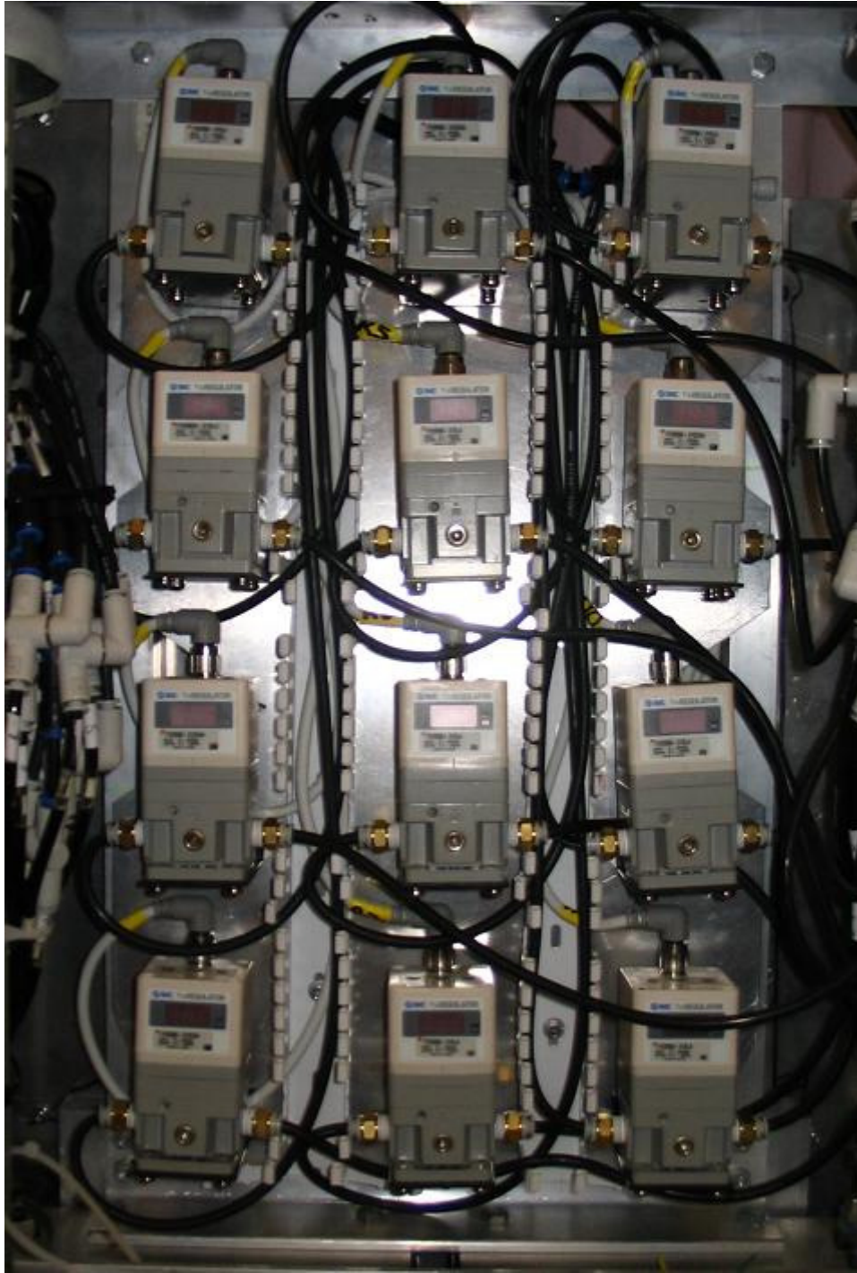
Figure 8: Regulator Valve Array
