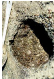
Figure 3. Stripping at Bottom of Hole (Washington 2005)
