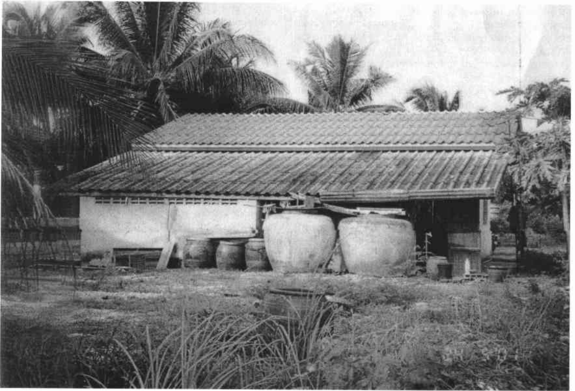
Fig. 1. Typical cement (large) and earthen (small) jars used in the study area for water use and storage. The 2 jars to the right are large (2,000 liters) and the 3 jars to the left are small (150 liters). The large jars are used for long-term water storage, whereas the small jars are refilled from the large ones for daily water use. Note the trough for carrying rainwater from the roof gutter into the large jars.
