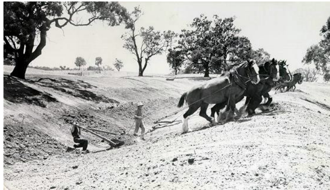
Fig. 1 Construction of the Wimmera-Mallee Domestic and Stock Channel System.
