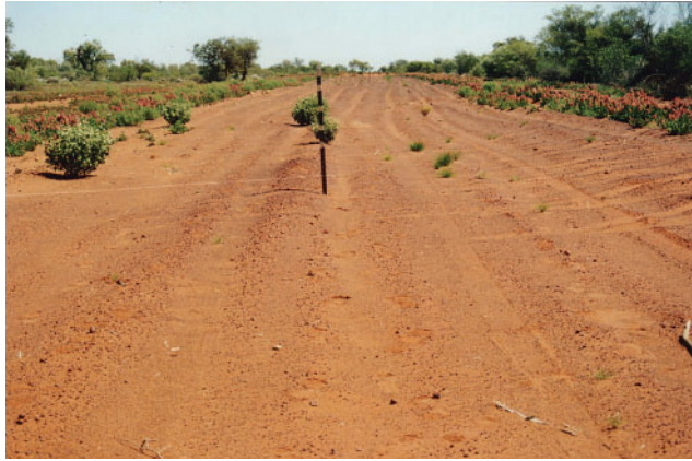
Fig. 6. Site 12A and B (Gillen Land System) 10 months after rehabilitation in 1992. The road remains bare, whilst Acetosa vesicaria dominates the verge. Note the relatively poor growth due to being overlain with sub soil.
