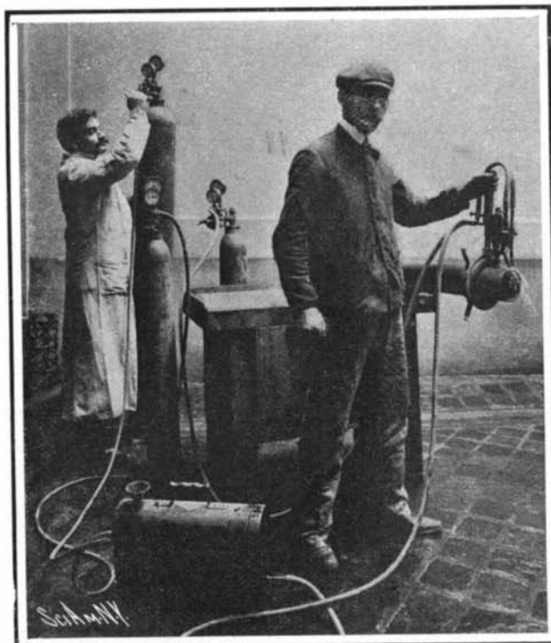
The Metal-Cutting Equipment.
