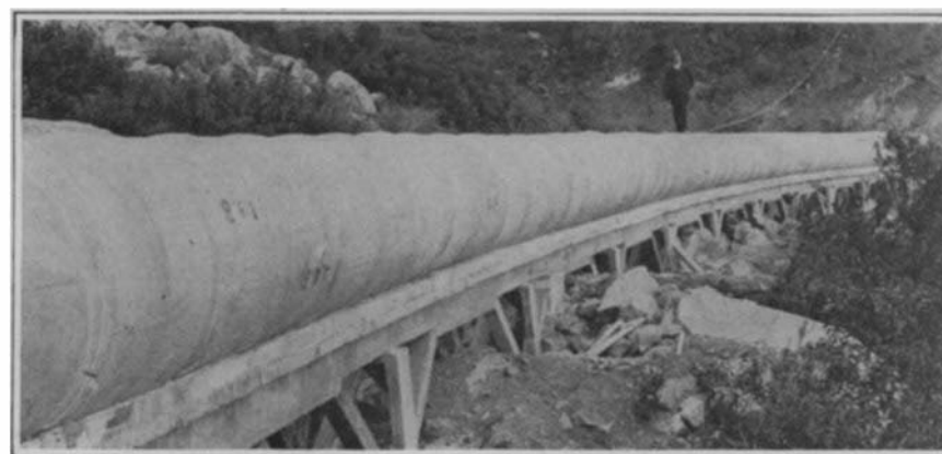
Forty-two-inch concrete siphon on the San Dieguito project
