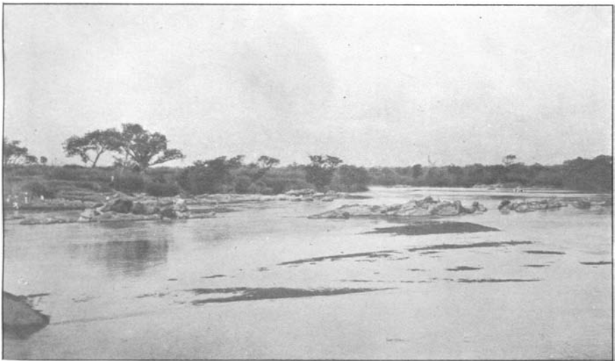
Fig. 2. View on the River Kaduna (during the dry season) at the point where it is crossed by the Baro-Kano Railway.
