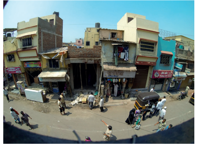
11:47:50 Laborers enter the construction site
