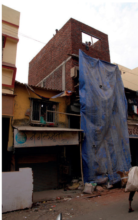
Figure 33 Protective tarp Protecting the street from construction as well as the construction from street view.
