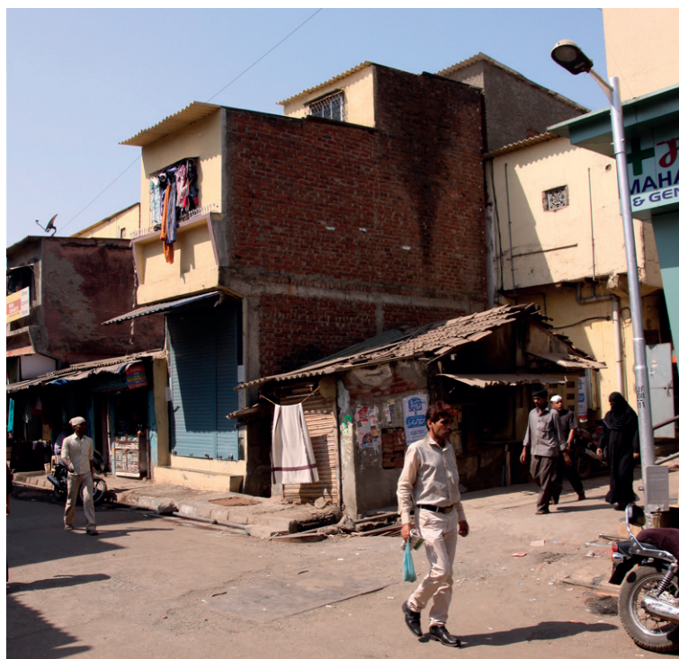
Figure 25 Individual development Uneven pace of development among unequal neighbours affects buildings which cannot follow the rhythm.
