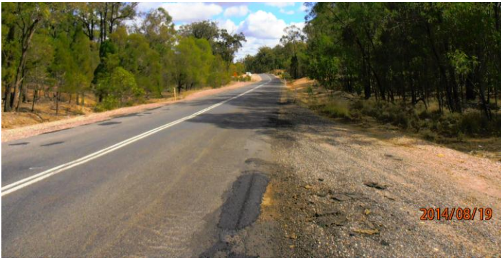
Figure 38: Dalby-Kogan road, taken on-site (King 2014).
