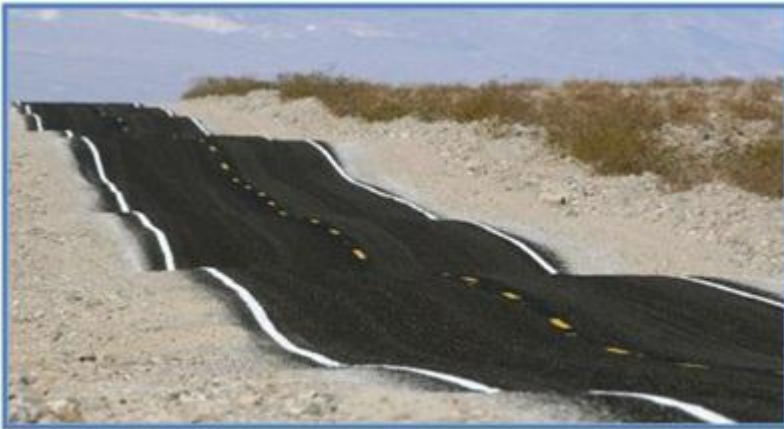
Figure 3: Rough Road Surface (California Department of Transportation 2014)
