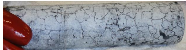
Figure 1 – ASR affected concrete sample
