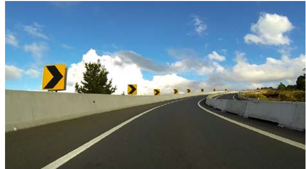
Figure 1 – Rigid central safety barrier with reduced sight distance
