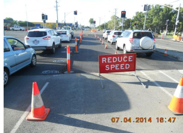
Figure 1 – Reconstruction occurring under traffic
