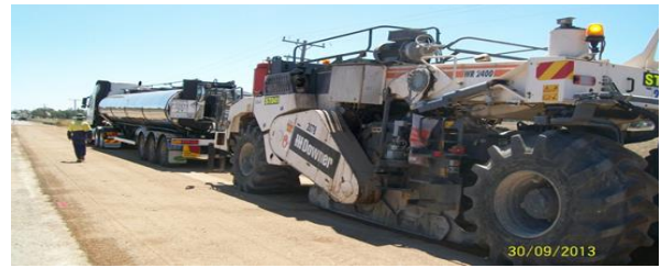
Figure 1 – In-situ Stabilisation using foamed bitumen on the Newell highway near Bellata
