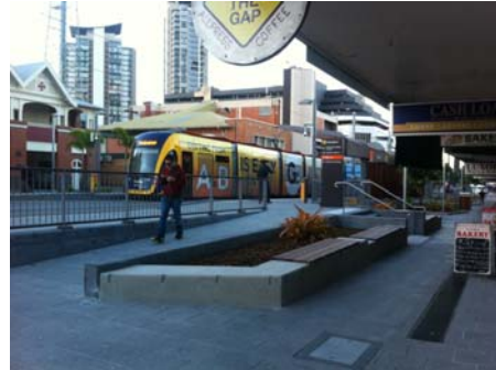
Figure 1 – Southport Light Rail Station 5
