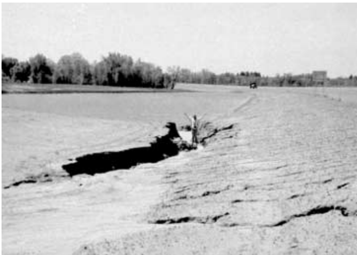
Significant erosion problems can occur during construction before new turf is established.
