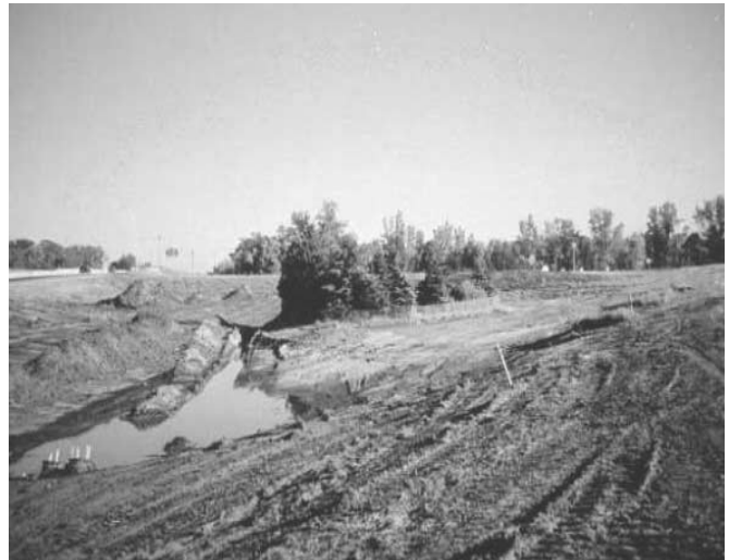
Protecting trees during construction
