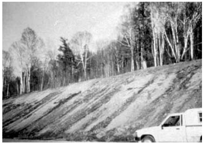
Significant erosion problems can occur during construction before new turf is established.
