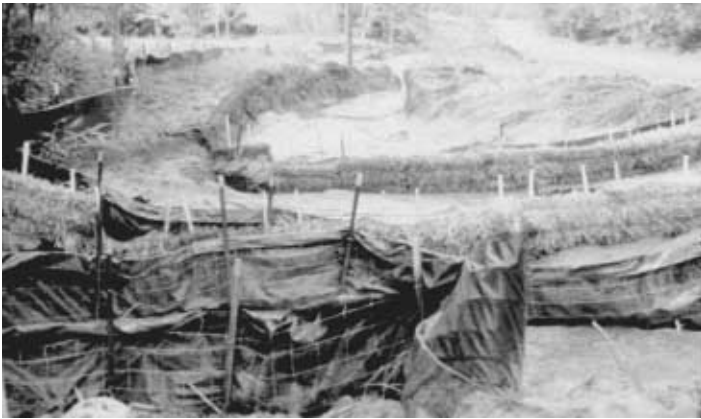
Use silt fence and hay bales to slow water velocity.
