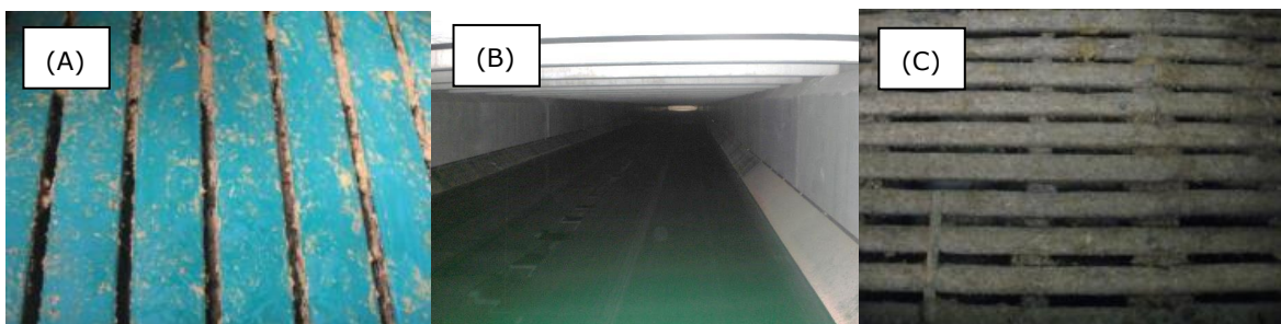
Figure 1 Measured floors. A) Traditional wooden slatted floor; B) "Groene Vlag" floor with C) V-shape belt.
