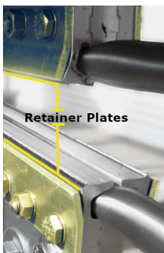
Figure 6: Functioned ‘G’ pattern RFJ with retainer plates
