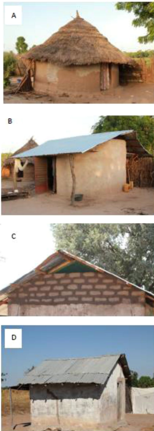
Figure 1. Types of study houses used in the mosquito survival experiments. Where (A) is a traditional thatched-roof house, (B) is a ventilated metal-roof house, (C) is a close-up of a screened window positioned in the gable ends of a ventilated house and (D) is a traditional metal roofed house without ventilation. Photographs by SW Lindsay.
