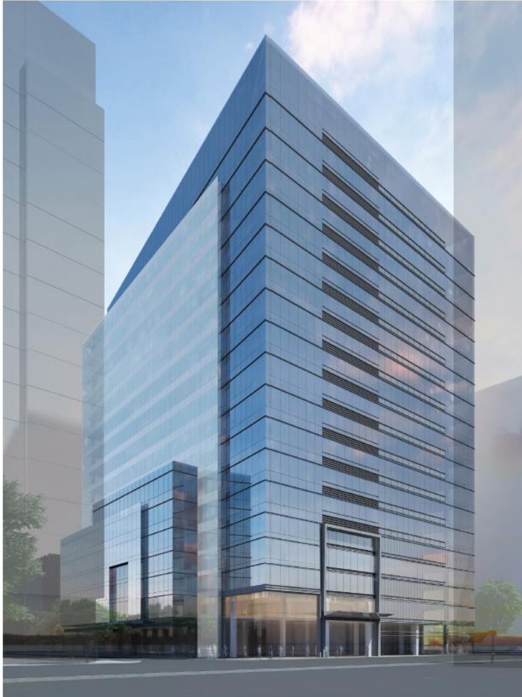
Figure 5. Image showing proposed Fan Pier Parcel I development. Note: From “Fan Pier-Parcel I” by The Fallon Company. (2013, June).
