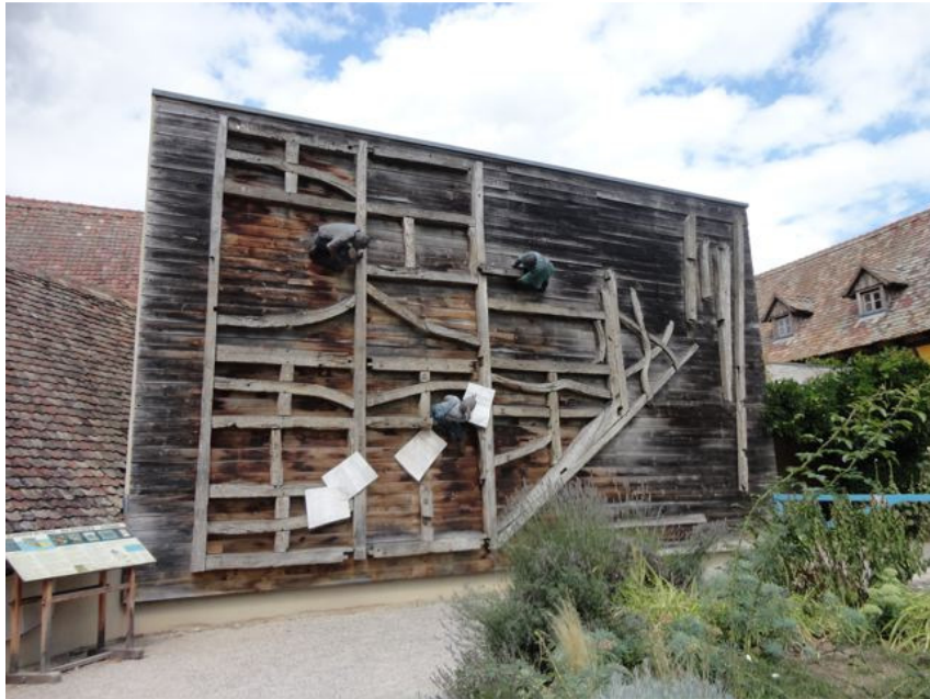
Figure 24: Ecomusée d'Alsace, Ungersheim. Pedagogical display explaining the making of a half-timbered house (first assembled horizontally and then propped up vertically)
