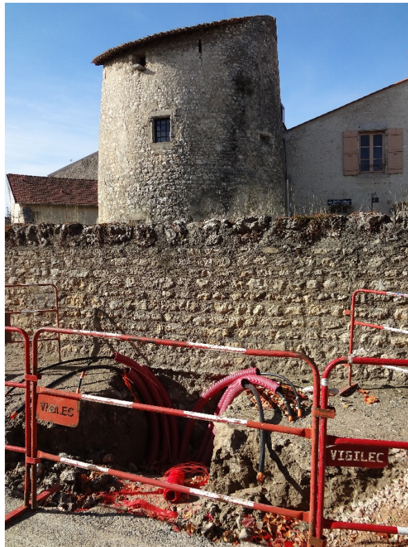
Figure 17: Burying electrical lines in Charroux (Auvergne)
