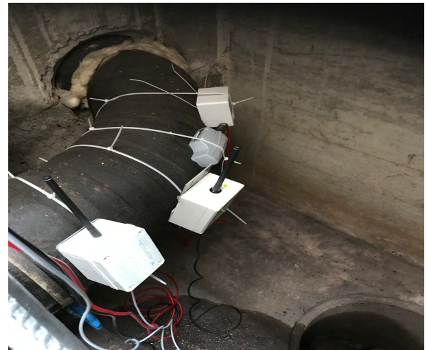
FIGURE 14. Synchronous LoRa mesh and LoRaWAN reference nodes in the service shaft in 3 m depth were mounted next to each other.
